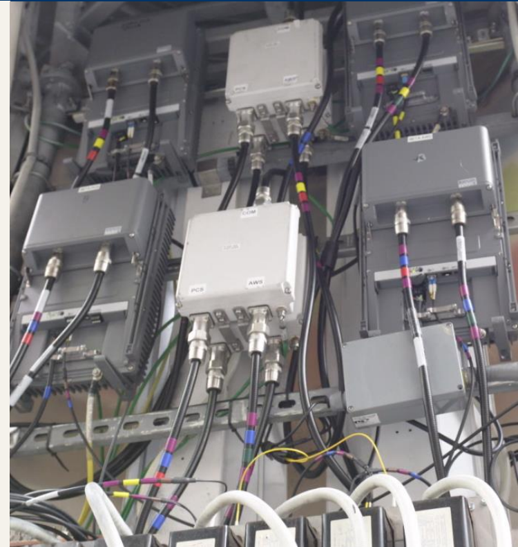
Small cell installation within a column
